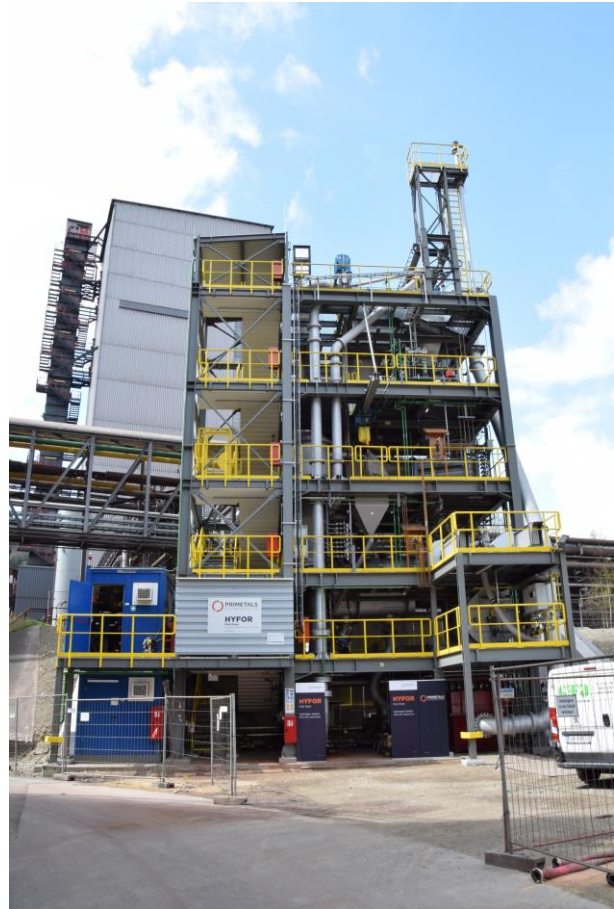
Fig. 1.: HYFOR pilot plant (copyright: primetals.com)
